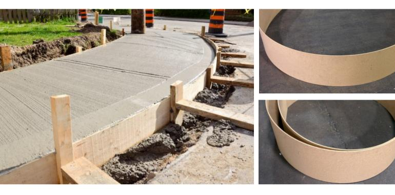
Benderboard is a hardboard product used for concrete forming applications, similar to lap siding. Benderboard is a thinner, lighter, less expensive option that bends easier (for a tighter radius) than most competing products.
