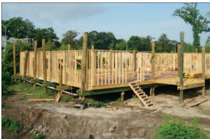
Round timber piling and glulam floor beams
