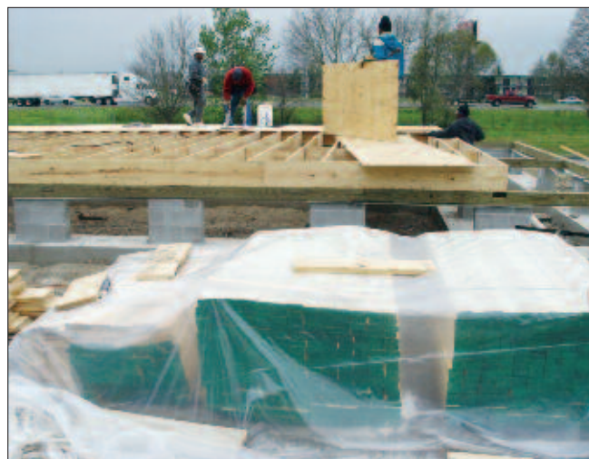
Proper job site storage
