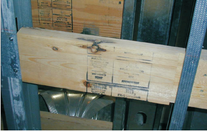
Pyro-Guard® is frequently used as blocking in the walls of Type I and II construction. Cleveland, OH.
