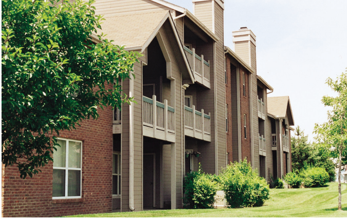
Sprinklers may be eliminated from balconies constructed of Exterior Fire-X®. Kansas City, MO.
