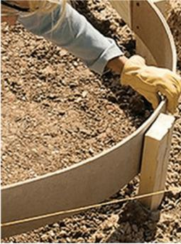
TruWood ValuForm flexible form boards are an engineered wood product designed for use in flatwork concrete forming applications. ValuForm installs easily and without special tools, providing time and labor savings when creating curved corners and intricate designs.
